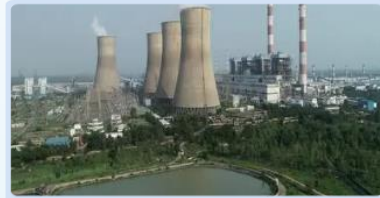
Power Plant RE Power
