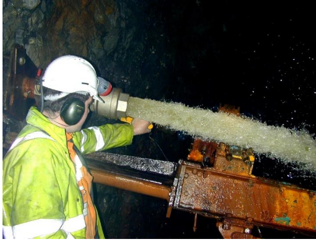
Monitoring of water ingress systems
