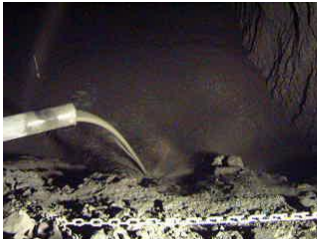
Paste Backfill being poured
